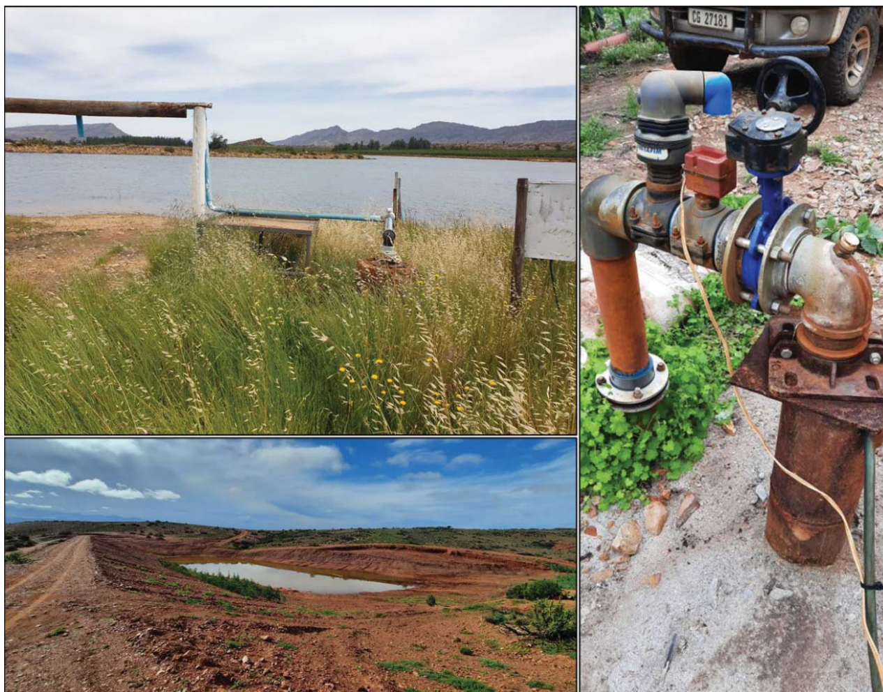
Figure 3-4 An example of a commercial farming groundwater supply scheme. (Top and bottom left) Boreholes are often used to augment storage in surface water bodies used for irrigation. (Right) Typical borehole infrastructure and headworks for irrigation supply.
