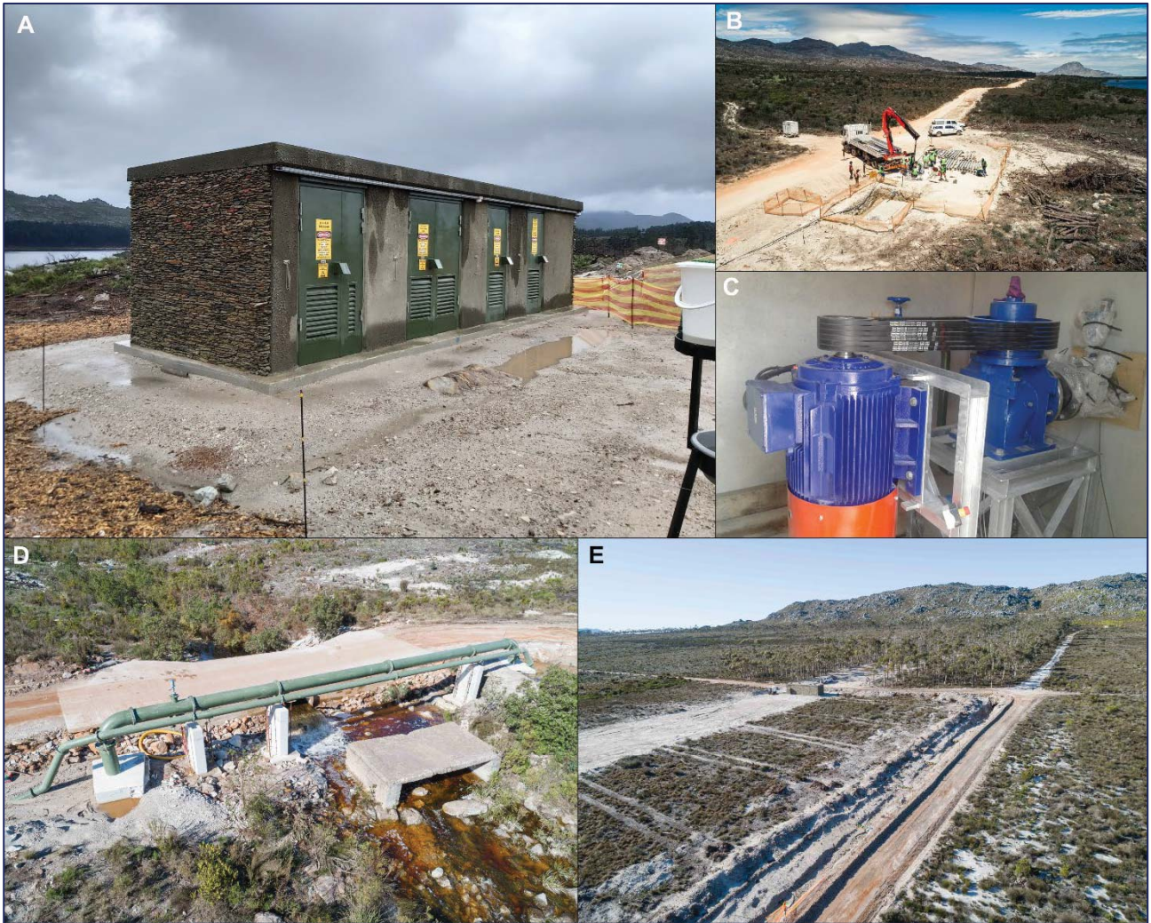
Figure 3-7 Example of a municipal bulk water scheme: The City of Cape Town Table Mountain Group Aquifers Steenbras Wellfield. A) Pump house structure. B) Installation of pump equipment during the construction phase by a contractor. C) Positive displacement pump installed at the production boreholes. D) Groundwater infrastructure pipeline (green) at a river crossing. E) Wellfield pipeline infrastructure development phase.
