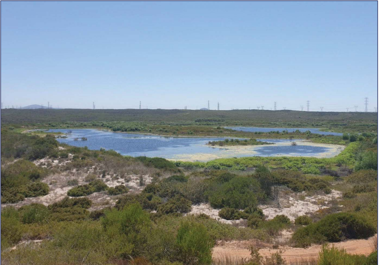
Figure 3-9 An infiltration basin where treated effluent is allowed to infiltrate into the aquifer through MAR, forming part of the AWRMS.
