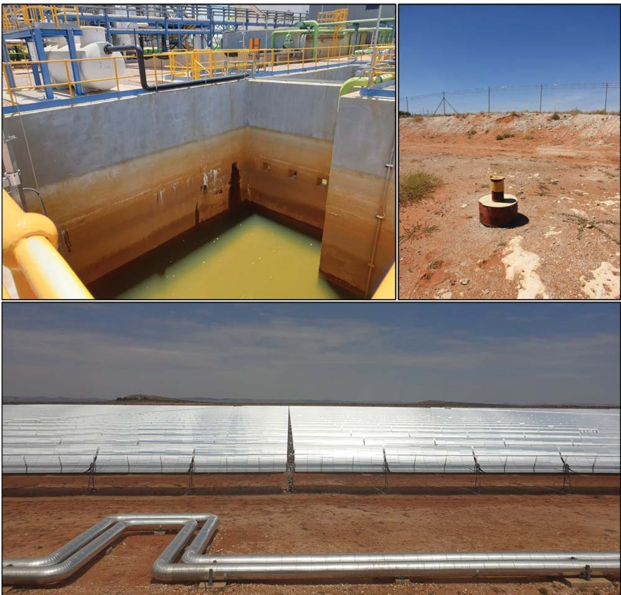
Figure 3-5 An industrial groundwater scheme where water is used in industrial processes, such as the generation of electricity using renewable solar energy. (Top left) Processed water is treated prior to discharge. (Top right) A monitoring borehole is shown in the foreground used for groundwater quality compliance monitoring. (Bottom) Array of solar panels used for generation of electricity.
